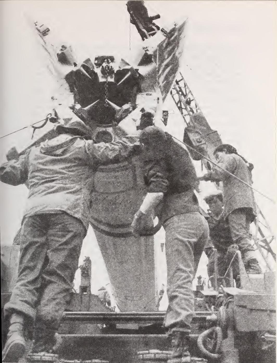
*Workers load a surface-to-air missile onto a transporter*
